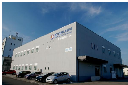
Elemental Technology Center
